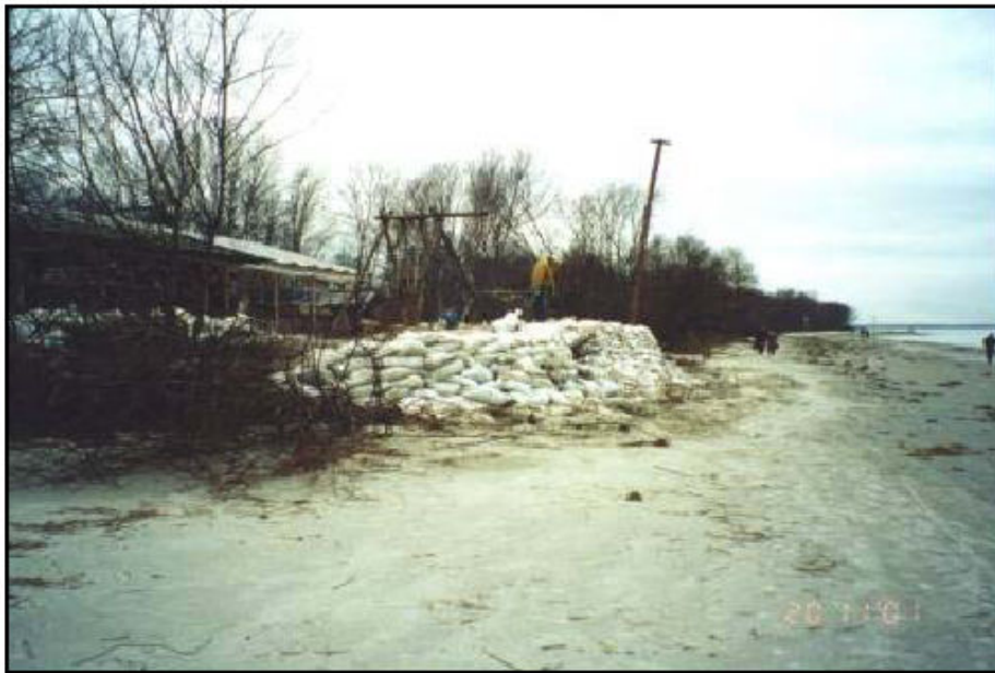
Fig. 8: Temporary defence measures in the place of the washed-off foredune. Jurmala, November 2001. Photo: G. Eberhards, November 2001. EUROSION Case Study
