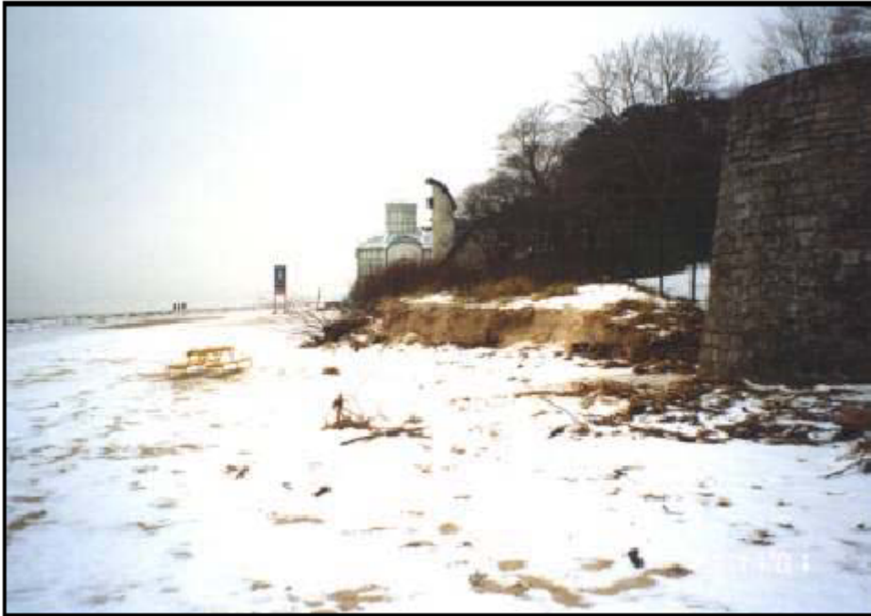
Fig. 9: Exposed recreation facilities after the storm surge erased the foredune. Jurmala, November 2001. Photo: G. Eberhards, November 2001.
