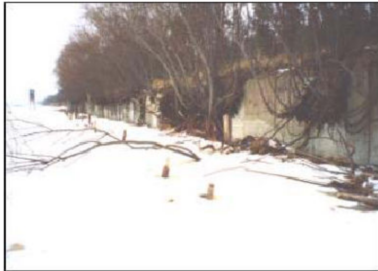
Fig. 7: The concrete base of the foredune, erected after the storm of 1969 and exposed again after the erasure of the foredune in November 2001. Photo: G. Eberhards, November 2001.
