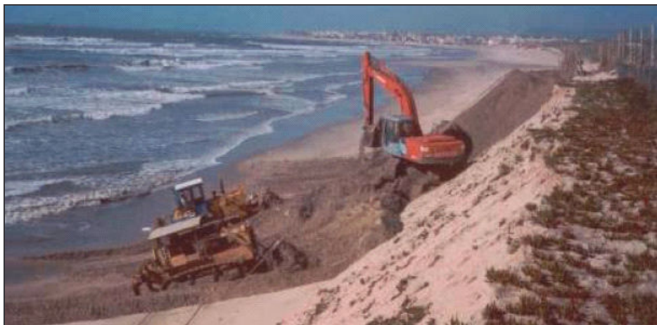
Figure 3: Sand ripping works near the 5 th hole, October 2000. (Source: Estela. EUROSION case study, at http://www.euroasion.org )
